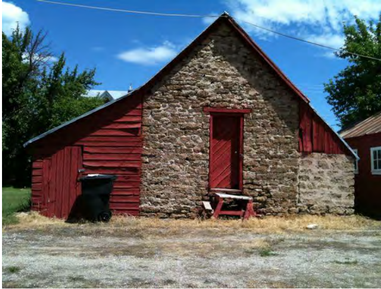
Granary west elevation. (Packer, 2010).
