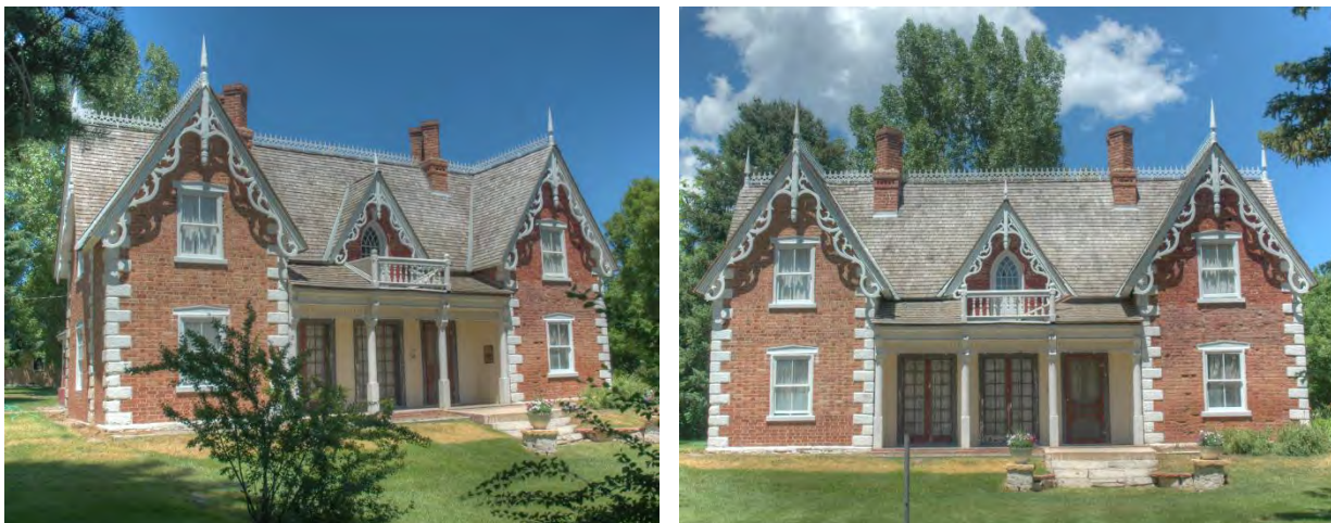
Watkins-Coleman House, view from southwest and south elevation. (Lobas, 2010).
