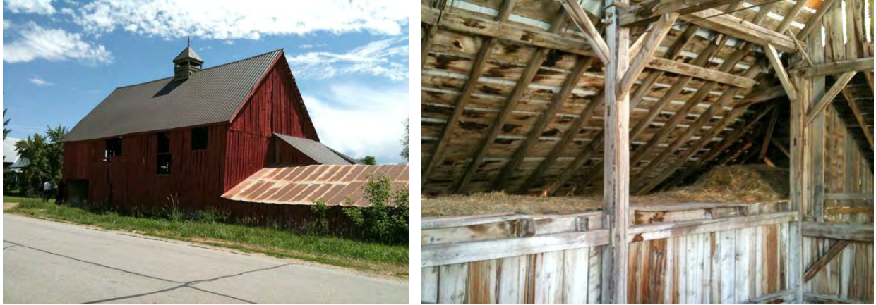
Barn, exterior view and interior showing post-and-beam structure. (Packer, 2010).
