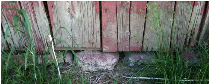
Barn foundation (cropped). (Packer, 2010).
